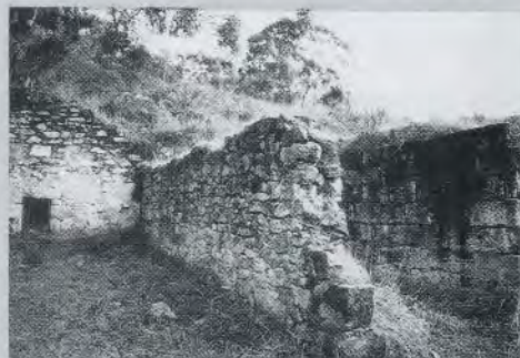
Enginehouse ruins with engine mounting block (right) and boilerhouse (left). Note the square opening to the underground flue at left.
