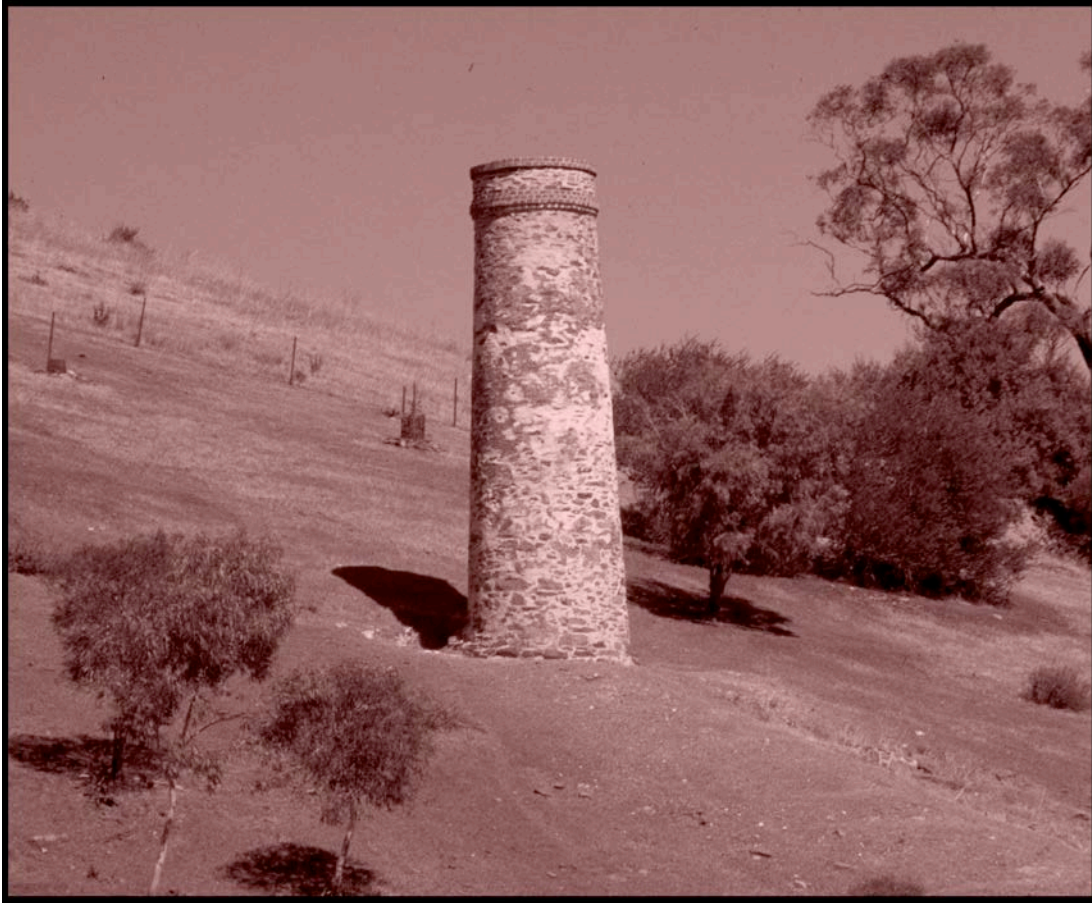
Figure 8: Glen Osmond smelter chimney.
