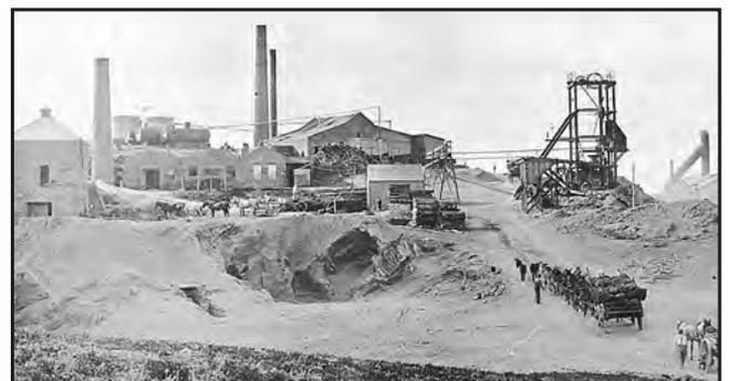
*Blinman Mine, c.1907. At right is the headframe at Main Shaft and at left is the two storey crusherhouse. (Photo 32763)*
