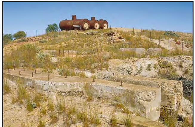
Remains of a circular buddle used to concentrate slimes from jigging machines. (Photo 43614)
