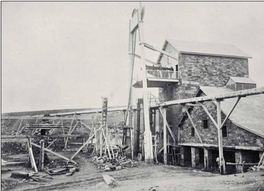
Morphetts Enginehouse, Burra Mine, 1875. This was erected in 1860 and contained an 80-inch beam engine. PIRSA Photo 035888.
